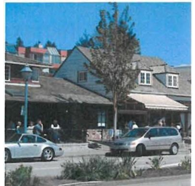
Varying building location with respect to set back will create outdoor seating opportunities
