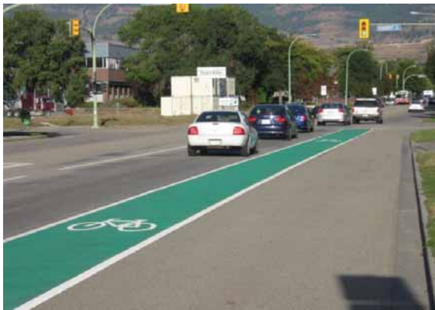
FIGURE 6.3.3 Photograph of Bicycle Lane Treatment, Kelowna B.C.
