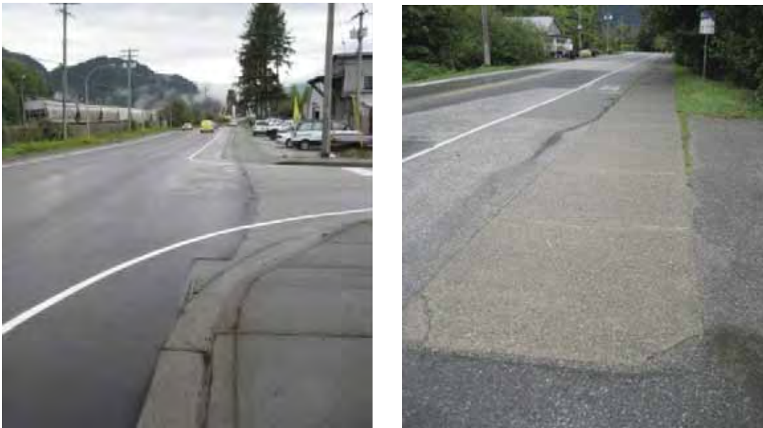
FIGURE 4.4.5 Photograph of Sidewalks, Buckley Avenue
