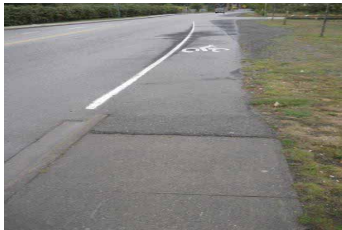
FIGURE 4.3.4 Photograph of Bicycle Lane, Buckley Avenue
