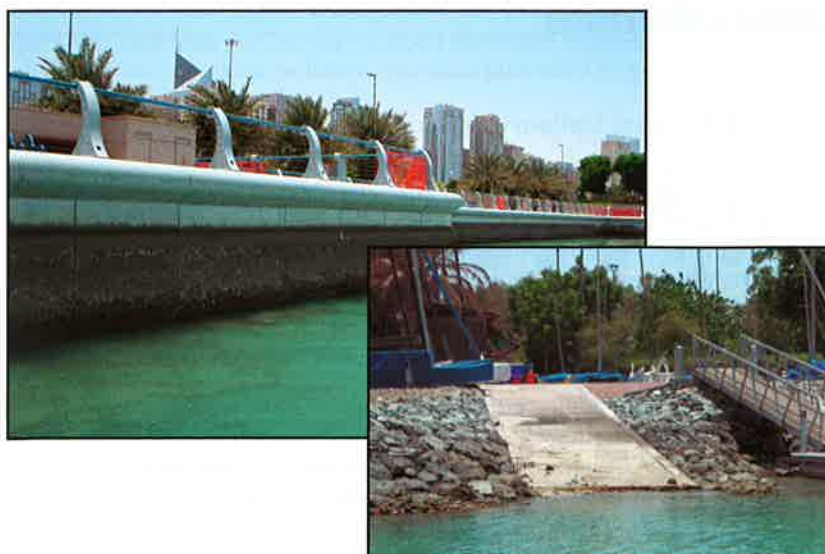
Figure 4.6 Solid Manmade Shorelines – Concrete Seawall and Boat Ramp
